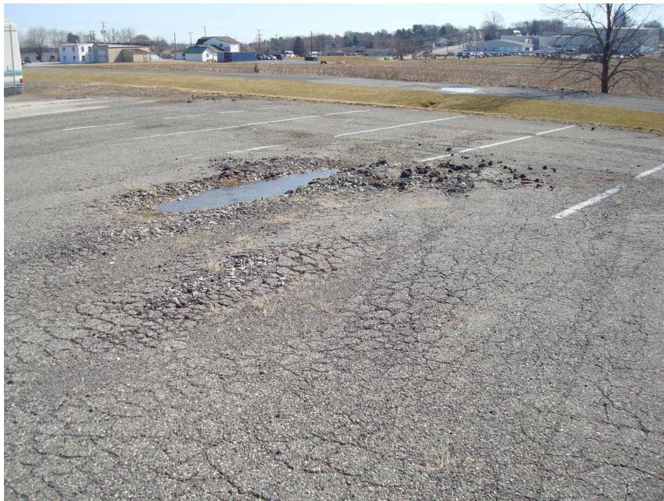
Pavement Cracking
